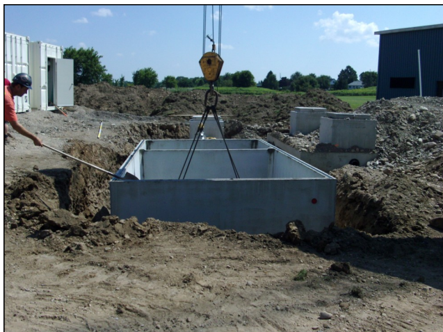
Erin District High School—System Under Construction
