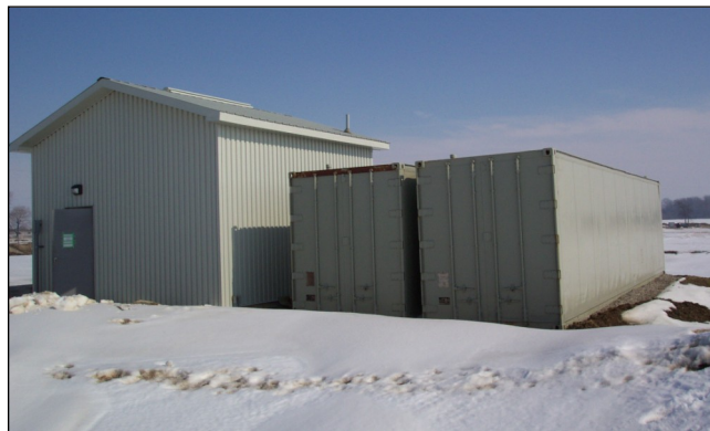
Building that houses the MS Filter is on the left and Waterloo Biofilter Treatment System shipping containers are on the right.
