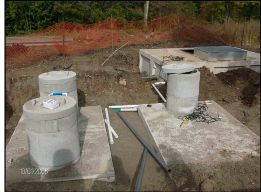
Septic and Treatment Tank Installation
