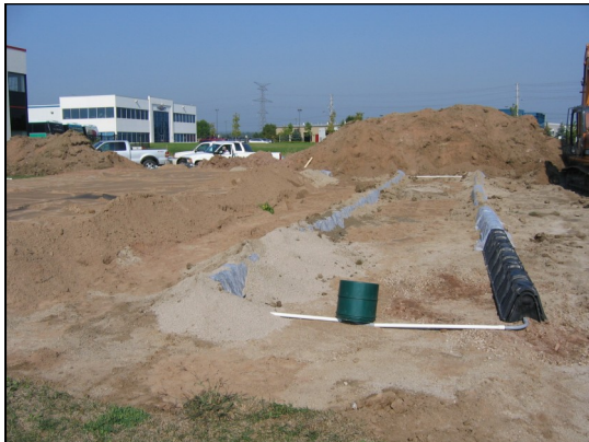
Shallow Buried Trench Disposal System
