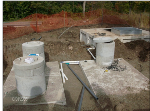
Septic and Treatment Tank Installation
