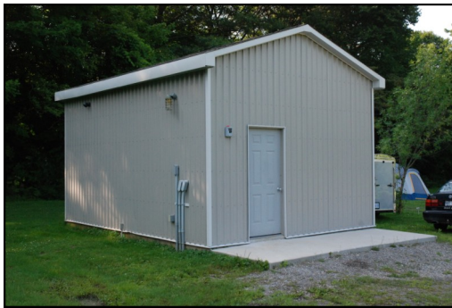
System Controls Building
