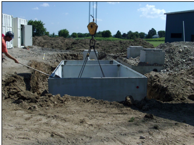
Erin District High School—System Under Construction
