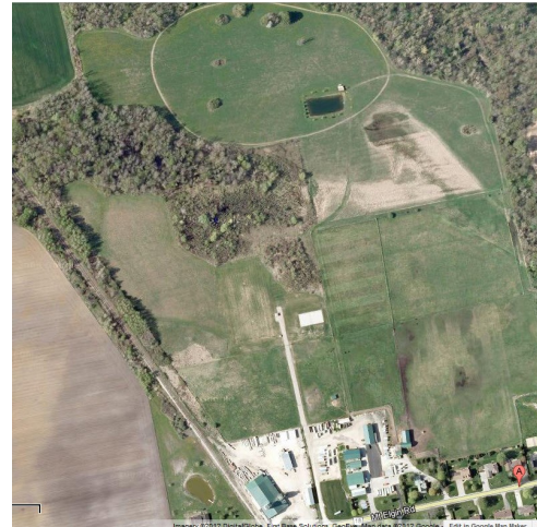
Mount Elgin WWTP
