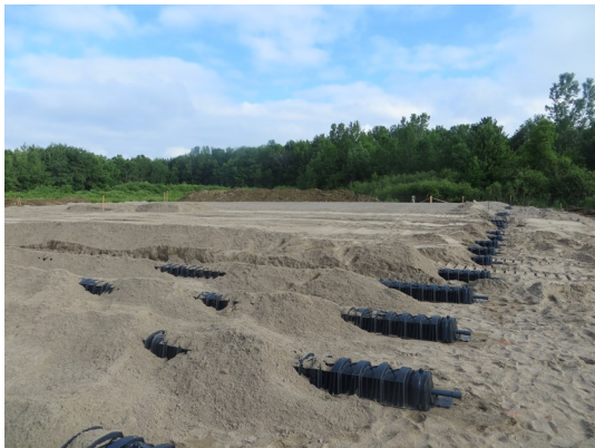
Construction of Shallow Buried Trench Disposal Bed
