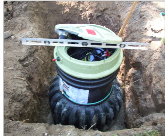
Installation of Environment One Grinder Pump Station
