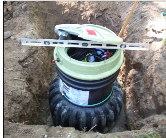
Installation of Environment One Grinder Pump Station
