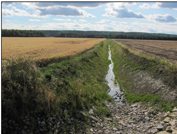
Drain Post Construction
